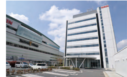
Food Safety Assurance Center (Namamugi Facility)
